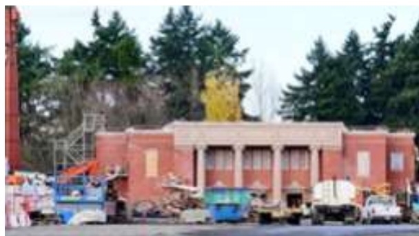
The Old Gym will be repurposed as an arts complex. The track has been removed to make way for classrooms which will be that level.
