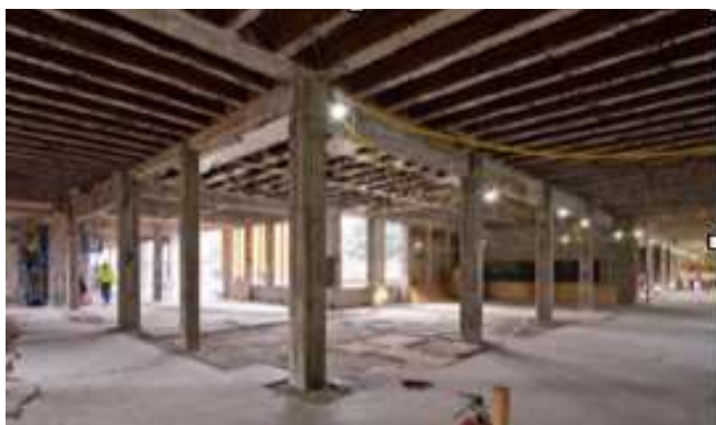
Demolition is nearly complete.
